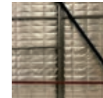
Foil Foam Insulation Reference Officeworks ceiling Photograph taken by Tyler Hill
